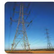
Electric Power Engineering
